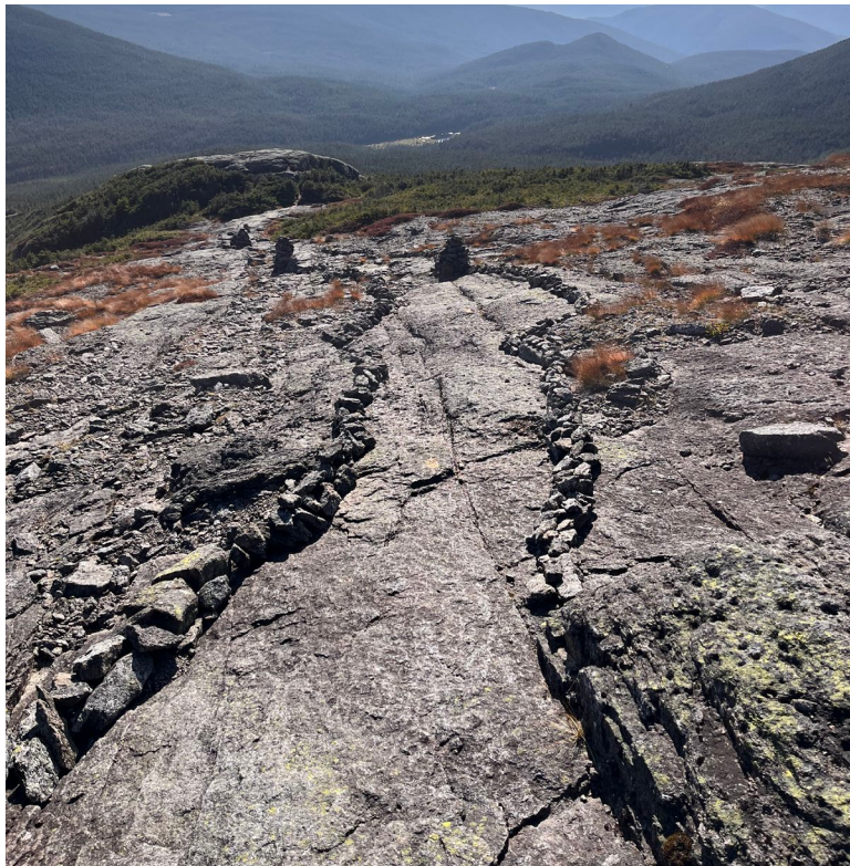
New scree wall on the back side of Marcy defining the trail
